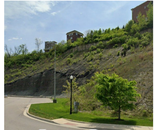
Steep hillside along Pavilion Parkway
