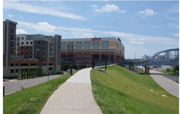
Elevated walkway trail along levee
